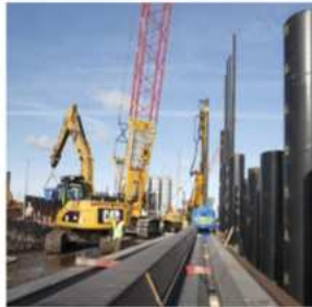
Quay job: Piling is now underway
